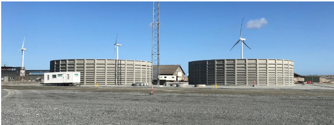
Figure 3 Water filtration - buffer tanks
